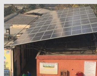
RAISED MOUNTING SOLUTION FOR SLS DAV SCHOOL, DELHI- 35KWp
